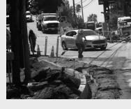
Ventura Blvd at a 90 degree angle. The sidewalk on the west side will be completed to comply with the American Disability Act. It will cross Fairway and connect with the sidewalk along the Coldwater Curve.
